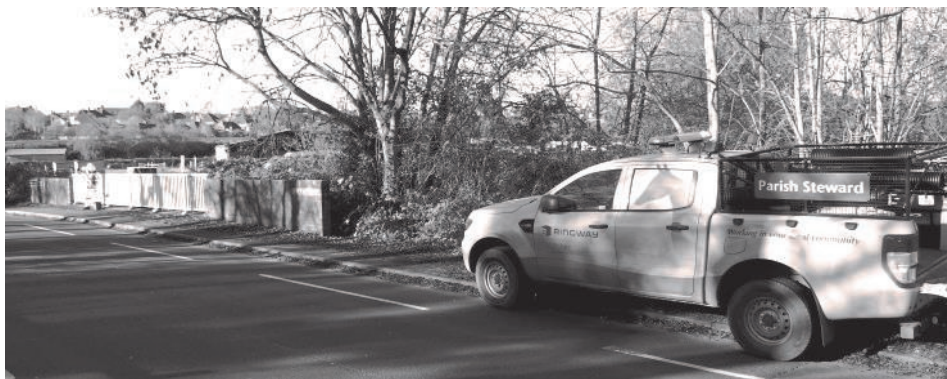
The parish steward has recently cleaned the green algae from the White Bridge in Laverstock .
