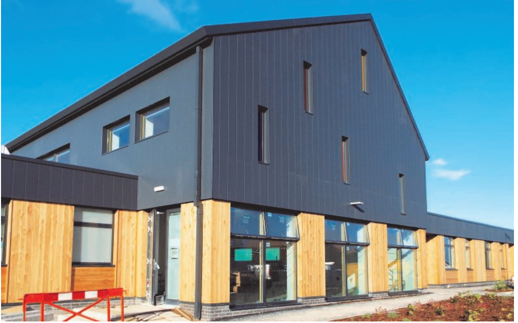
The new school building pictured in the week before hand-over
