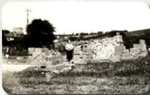
Photo 3: Barbara standing in the foundations of her new house in Potters Way - private collection.
